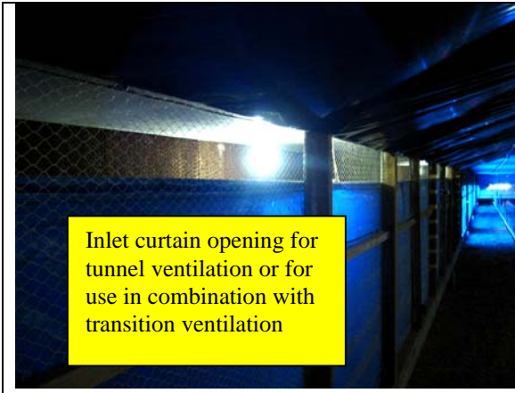
Photo 4. View of the air inlet curtain from the inside of the house. Observe that 4 fans are running at the end and this is the maximum opening allowed for proper house pressure. Opening of the inlet curtains can be relative small and proper airspeed again should be 900 fpm in a 40 f (12 m) wide house.
